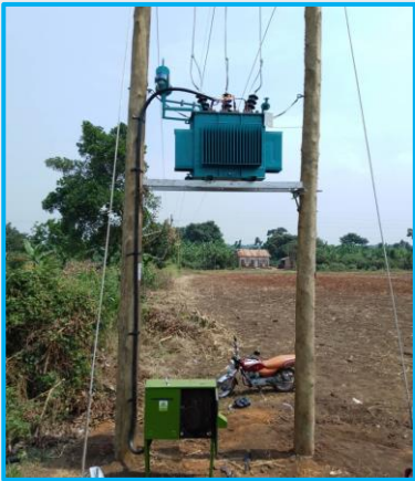
MV Line Construction and Maintenance
