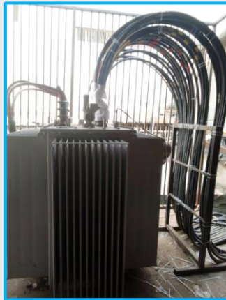
General Transformer Maintenance
