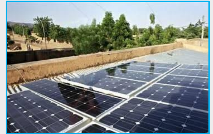
Solar Installation Works and Maintenance
